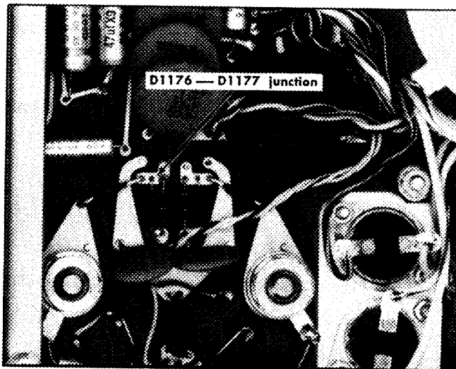
Fig. 6-4. (a) Power supply input voltage measuring test points. (b) Test oscilloscope probe connection.
